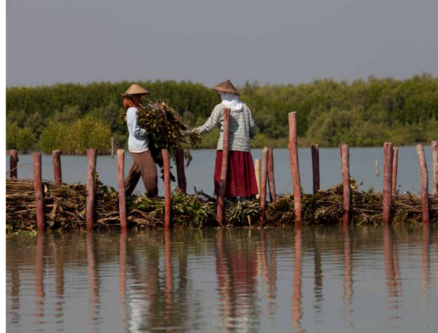
The local community helped build permeable structures in Demak, recompensed with financial support and training for new local economic activities.
