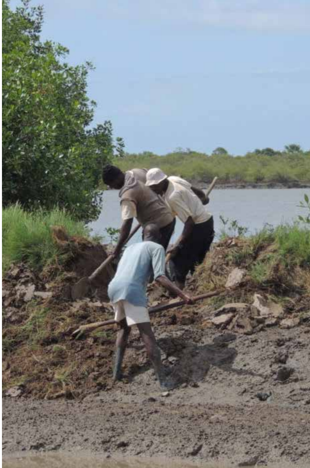
In Guinea-Bissau, local farmers helped break dikes to restore hydrology for ecological mangrove restoration.
