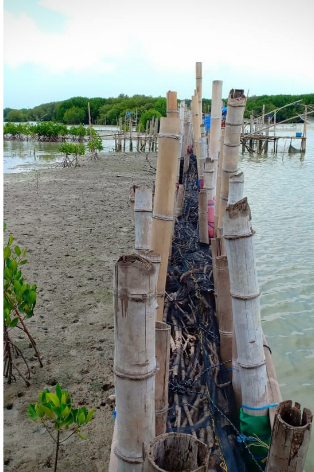
Permeable structure that traps sediment to stabilise the coastline at Bogorame Timbulsloko village, Java.
